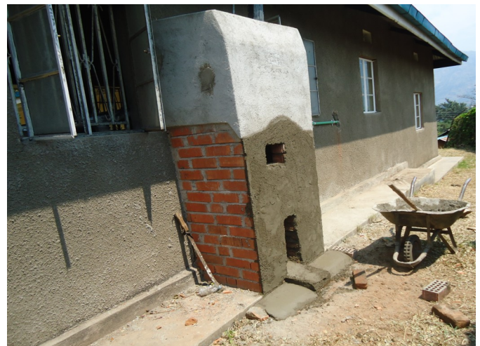
The combined water heater and incinerator designed by Richard Kizito.
