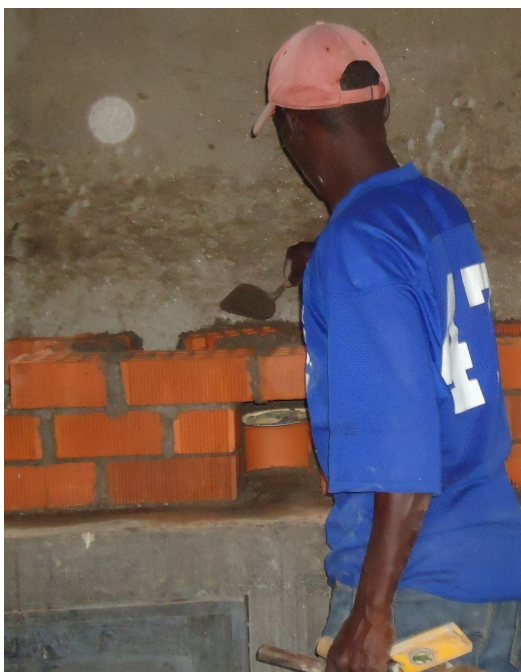
Richard Kizito at work on building the stoves.
